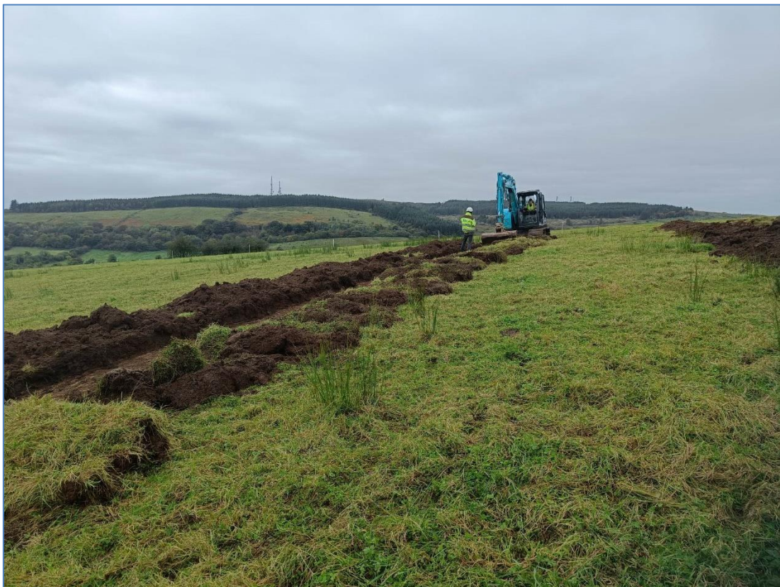
Plate 6: Ongoing test excavations at Glennagross.
