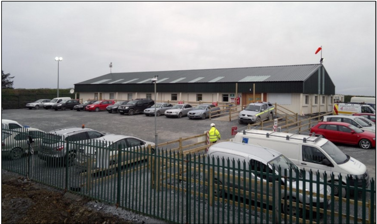
Figure 4-2: Typical temporary site construction compound on a wind farm
