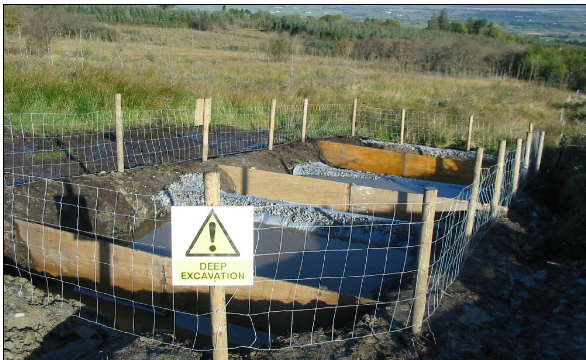
Figure 4-5: Typical Three-tiered Settlement Pond with Stone Filter
