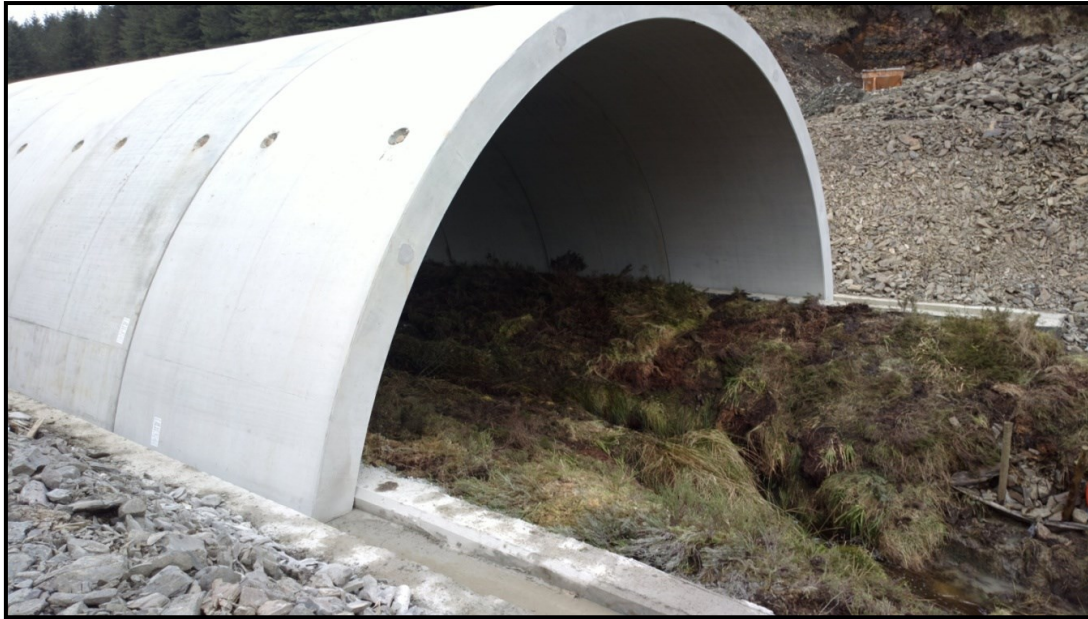
Figure 5: Typical clear span pre-cast concrete units in place over an existing watercourse
