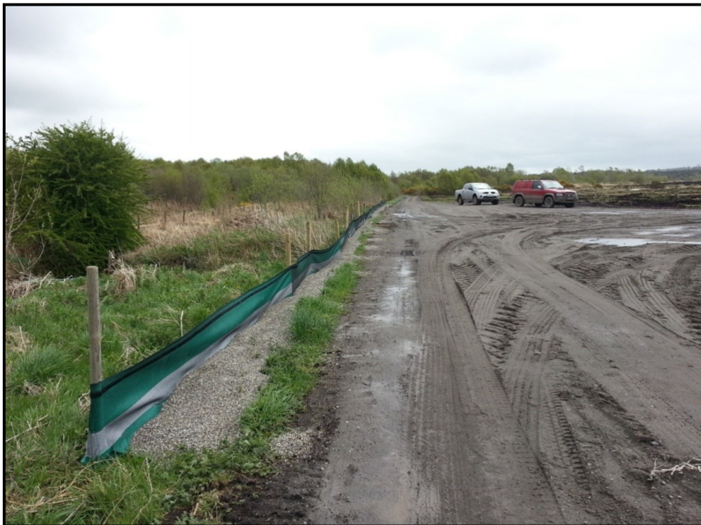
Figure 8: Silt curtain containment along existing tracks near watercourses
