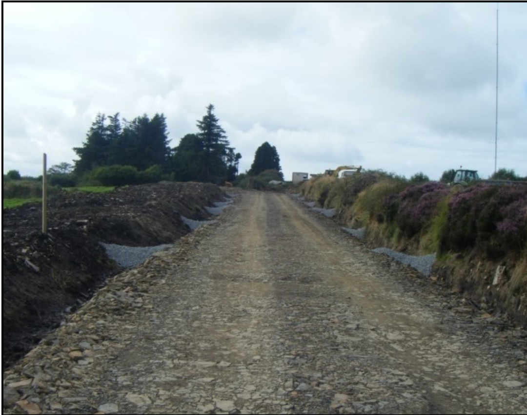
Figure 11: Examples of check dams along trackside drainage channels
