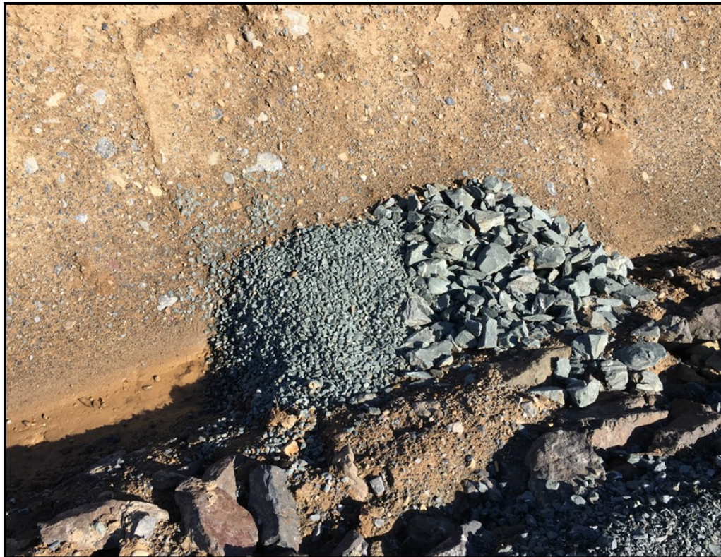
Figure 9: Stone check dam with large aggregate on downstream side
