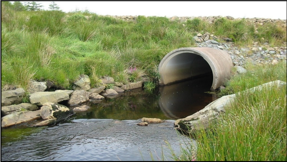
Figure 6: Typical concrete pipe channel crossing
