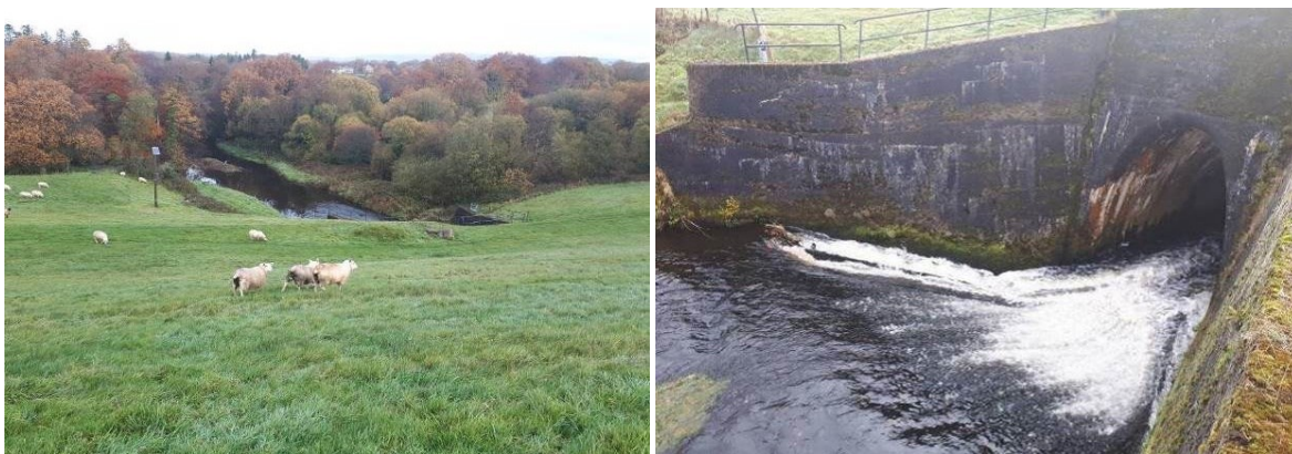
Plate 17: The intersection of the Blackwater River and the headrace of Ardnacrusha Hydro-scheme (left). Upper end of the culvert for the Blackwater River under the headrace of Ardnacrusha Hydro-scheme (right).
