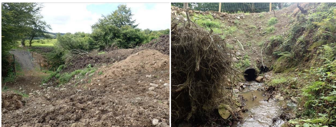
Plate 29: Denuded area adjacent to the North Ballycannan Stream (left). Instream disturbance (right) within the corridor of the North Ballycannan Stream (right).
