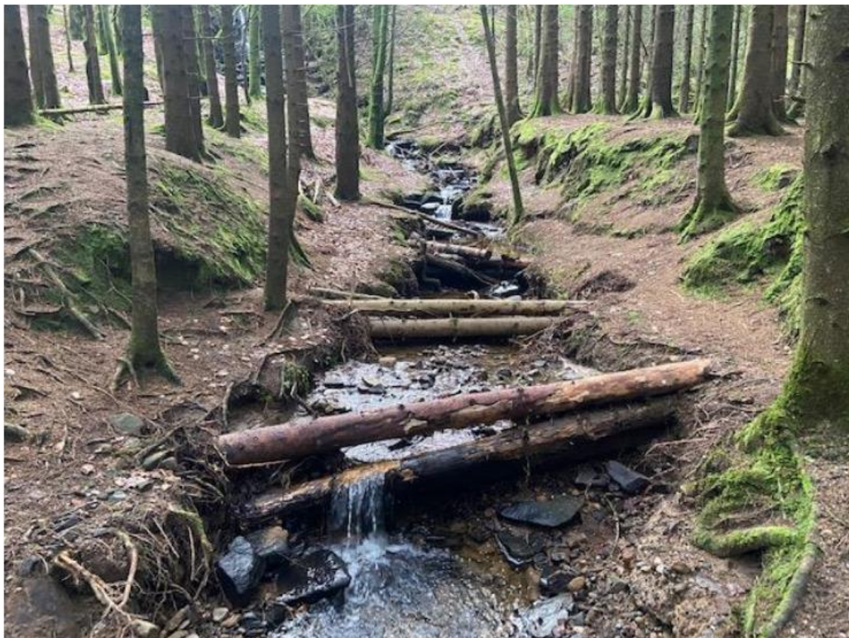
Plate 3: Example of a stream/drain partially blocked to slow the flow and limit erosion/soil loss.
