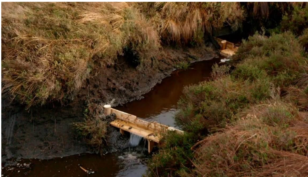
Plate 1: Series of partial blocking along drain of high gradient.
