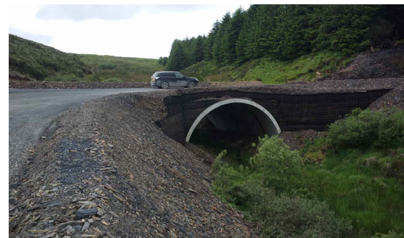
Bottomless Arch Culvert Crossing
