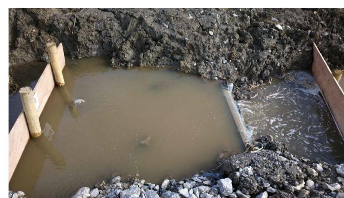
Baffle/Weir Detail
