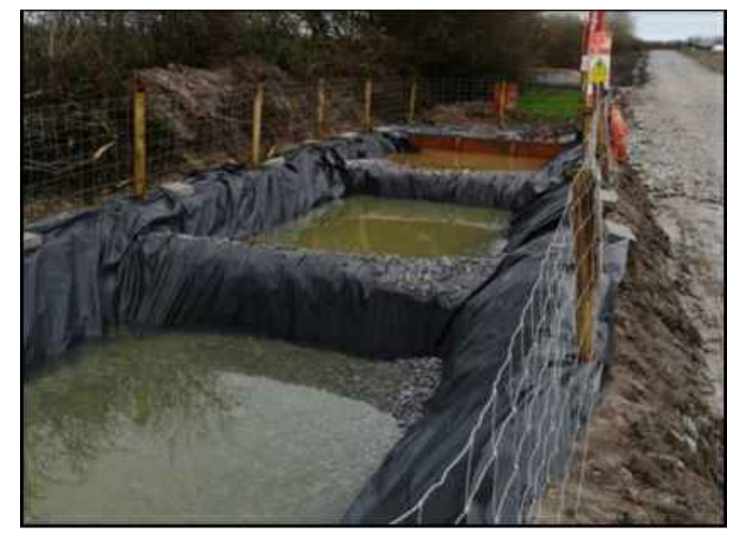
Completed Settling Pond System
