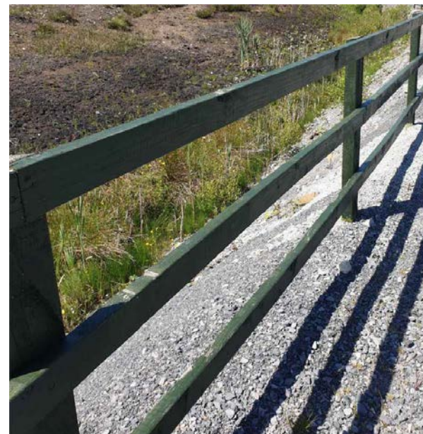
Timber Post & Rail Fence Detail
