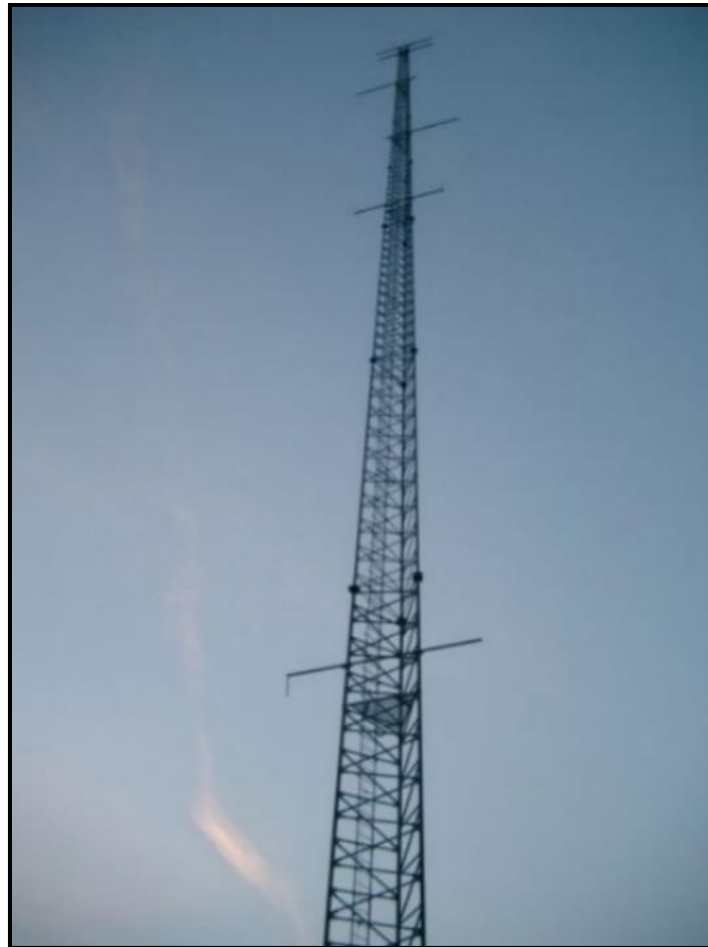
Figure 2-8: Meteorological mast on a wind farm
