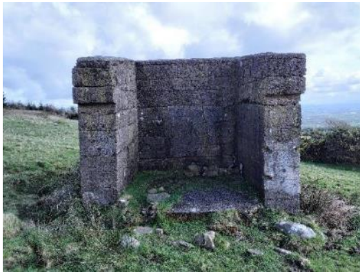
Plate 18: Stone structure present within the proposed wind farm site displaying 'negligible' suitability for roosting bats
