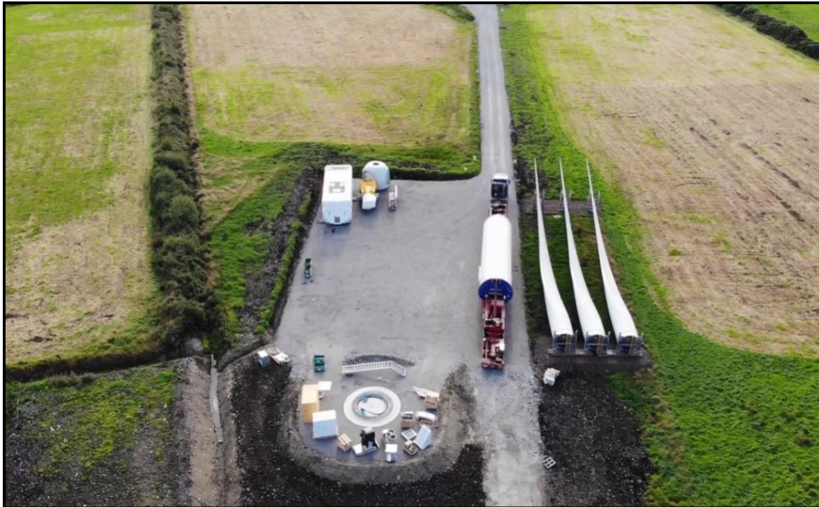
Plate 10. Example of typical finished hardstand on a wind farm.
