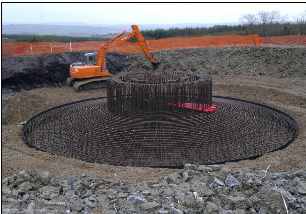
Plate 9. Typical construction of a wind turbine base.
